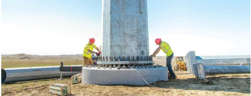
Work is progressing on setting the steel towers on the concrete foundations for the North Killdeer Loop transmission project. There are 161 structures being set in total.
