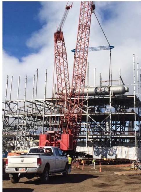
The 250-ton pool reactor is set in place as part of Dakota Gasification Company's urea facility construction project.
