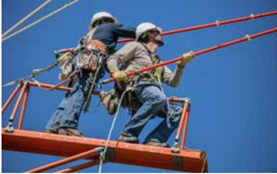
Hot sticks allow Basin Electric line workers to work on energized transmission lines.
