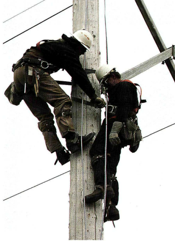
Leon Conitz (right) plays the part of an injured lineworker as Perry Kress prepares to lower him to safety during a pole rescue exercise. Conitz and Kress are journeyman lineworkers with Basin Electric TSM.
