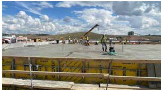
Concrete being poured near Dry Fork Station.
